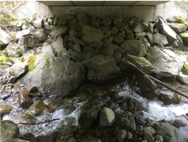
Left Bank Abutment when facing downstream
