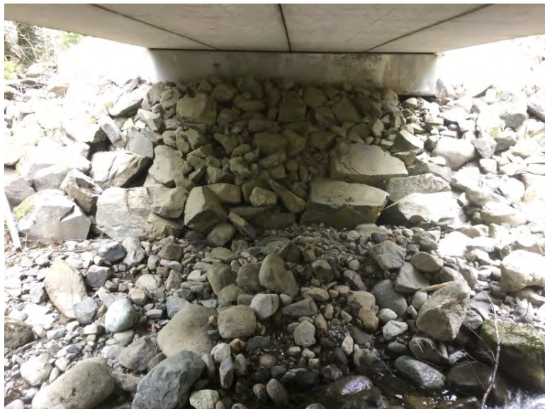
Right Bank Abutment when facing downstream
