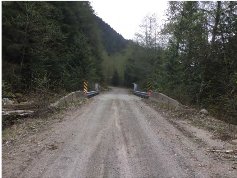
Approach from Right Bank when facing downstream
